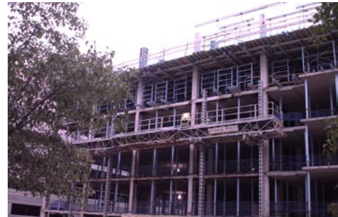
Scaffold System for Masonry Installation
